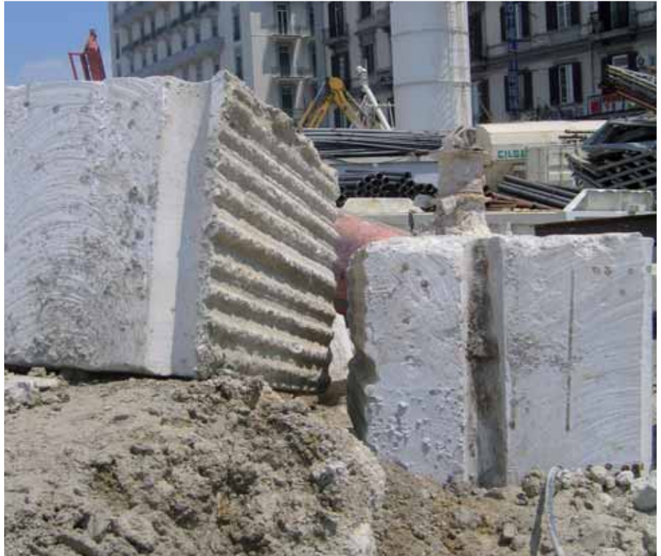
“Concrete-to-concrete joint” obtained by partial overlapping between primary and secondary panels.
